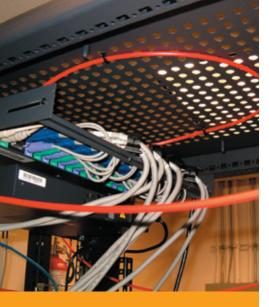
Firetrace does not occupy valuable rack space. This red Firetrace Detection Tubing can be run unobtrusively across the top of the rack.
